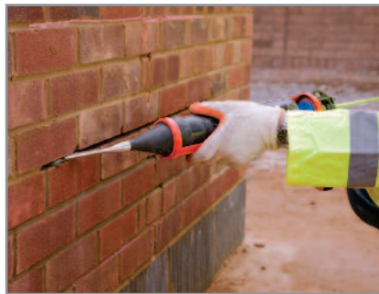
5. Inject into the slot or hole in a continuous operation. Typical working life of the mixture in the pail is around 2 hours with re-agitation . The cartridge should be emptied within 5 minutes. If the injection process is interrupted for any reason, empty any cartridge contents back into the bucket and re-mix until it again reaches a smooth injectable consistency
