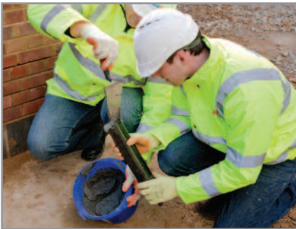
4. Check the piston is a snug fit in the cartridge and adjust in accordance with the pointing gun instructions. Load the mixture into the cartridge in the pointing gun immediately after agitating
