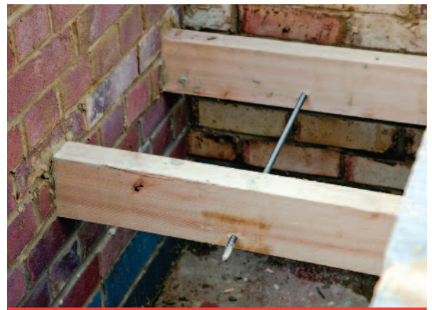
BowTie HDs installed through parallel floor joists
