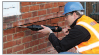
3. Using the Helifix Pointing Gun, inject a bead of HeliBond along the back of the slot
