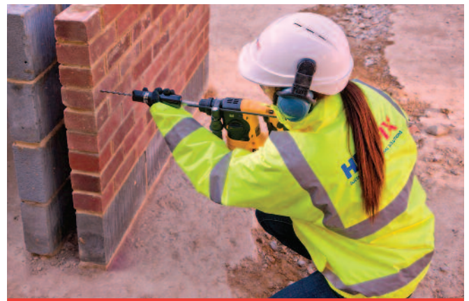
DryFix tie being power-driven into pilot hole
