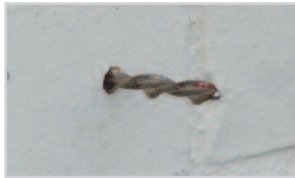
1. Install tie into inner or outer leaf masonry
