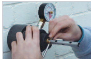
4. Place the cross pin through the LTK and take up the slack on the central nut
