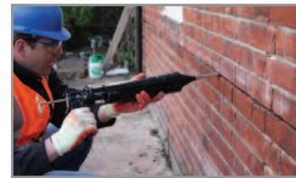
5. Insert a further bead of HeliBond over the exposed HeliBar, finishing 12mm from face and 'iron' firmly into the slot using the HeliBar Insertion Tool
