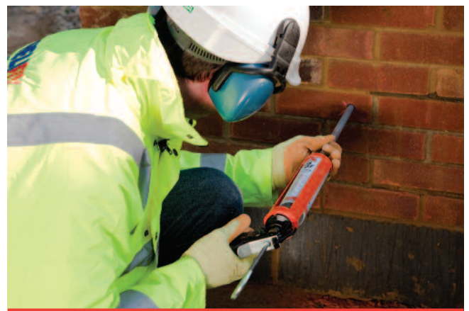
Injecting EpoxyPlus resin into near leaf to complete the ResiTie installation
