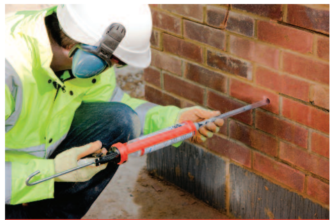
Injecting resin to complete the RetroTie installation
